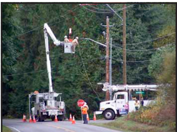
System upgrade along Prospect Ave
