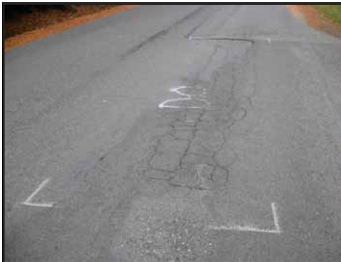
*Pavement area identified for "digging out" in advance of new asphalt overlay.*
