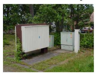
around the phone company infrastructure site just outside the gate. The several "boxes" located there comprise what technicians call an "RT" (short for remote terminal) which serves as one of two central equipment locations for the electronics connecting Qwest networks with individual homes
